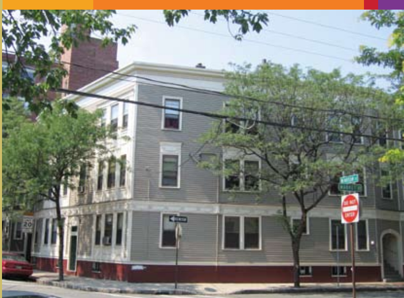
Homeowner's Rehab, Inc. acquired, renovated, and preserved the affordability of 95 family-sized rental units scattered throughout the Wellington/Harrington and Area IV neighborhoods, including this 9-unit apartment building which was renovated in 2002.
