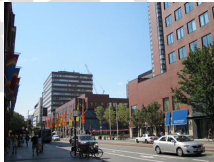
view from MIT/Kendall station looking towards the Cambridge Center Area
