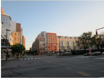
view along Third Street looking towards the Volpe site
