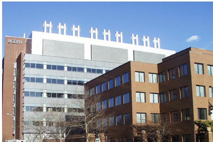
The Biogen building in Kendall Square partially expresses the mechanical equipment and partially screens it (Biogen, Cambridge)
