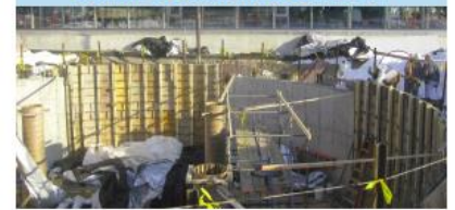
Example of Storage Tank Construction
