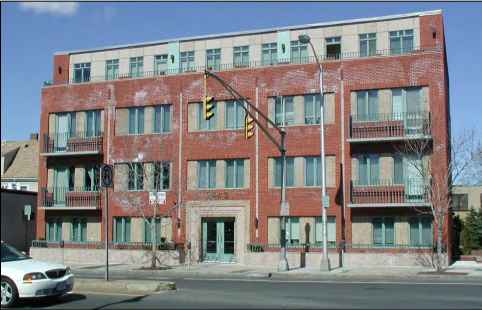
Example of a residential development on North Massachusetts Avenue built under current zoning – Approx. 45 feet
