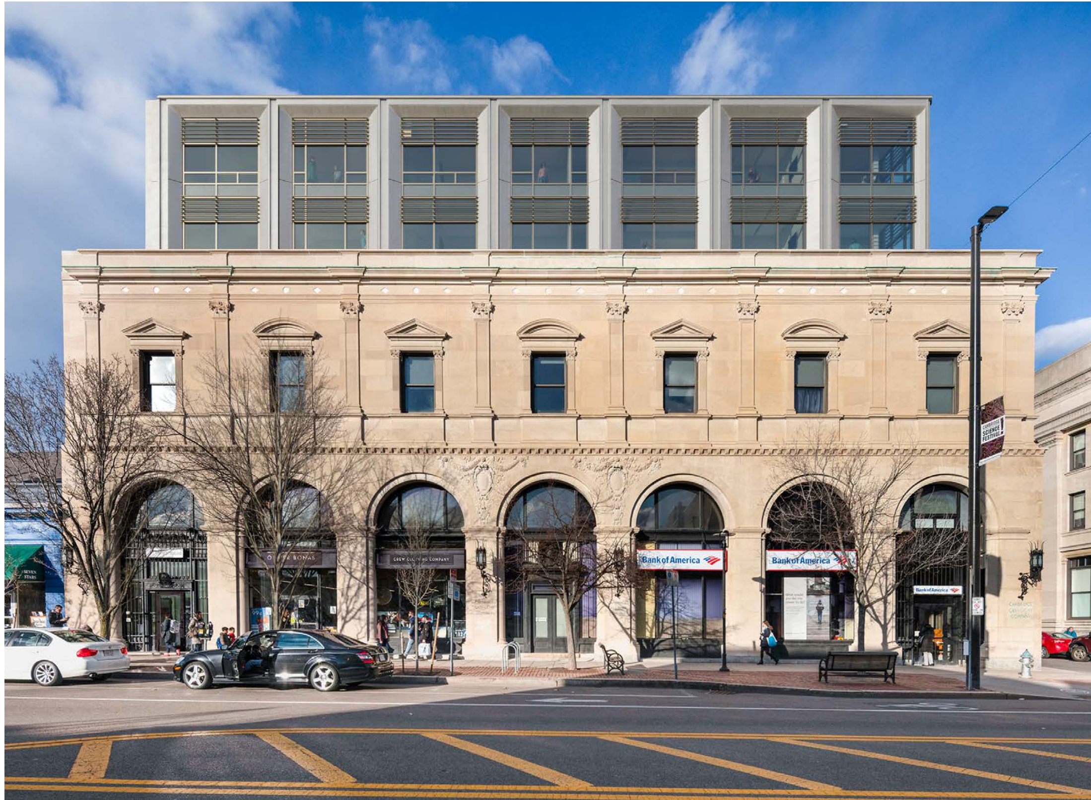
1B View from Massachusetts Ave Looking North
