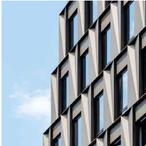
Unitized Curtain Wall with Vision Glazing
