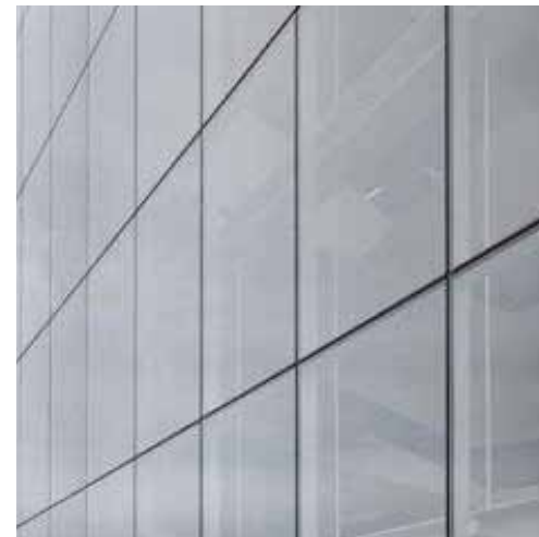
Structural Silicone Glazed (SSG) Curtain Wall System
