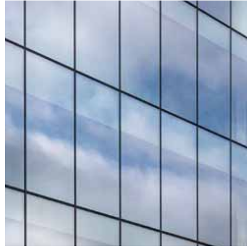
UNITIZED CURTAIN WALL WITH VISION AND SHADOW BOX GLAZING (PIER 4 OFFICE BUILDING)
