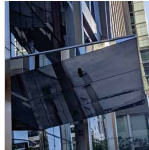
METAL CANOPY (MASS MUTUAL OFFICE BUILDING)
