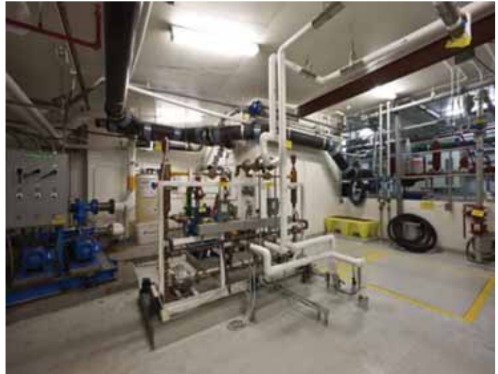
Figure 21. Image of blackwater treatment system in NYC project – Courtesy of Natural Systems Utilities
