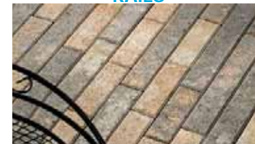
PERMEABLE UNIT PAVERS - TYPE 1
