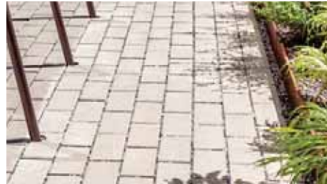
PERMEABLE UNIT PAVERS - TYPE 2
