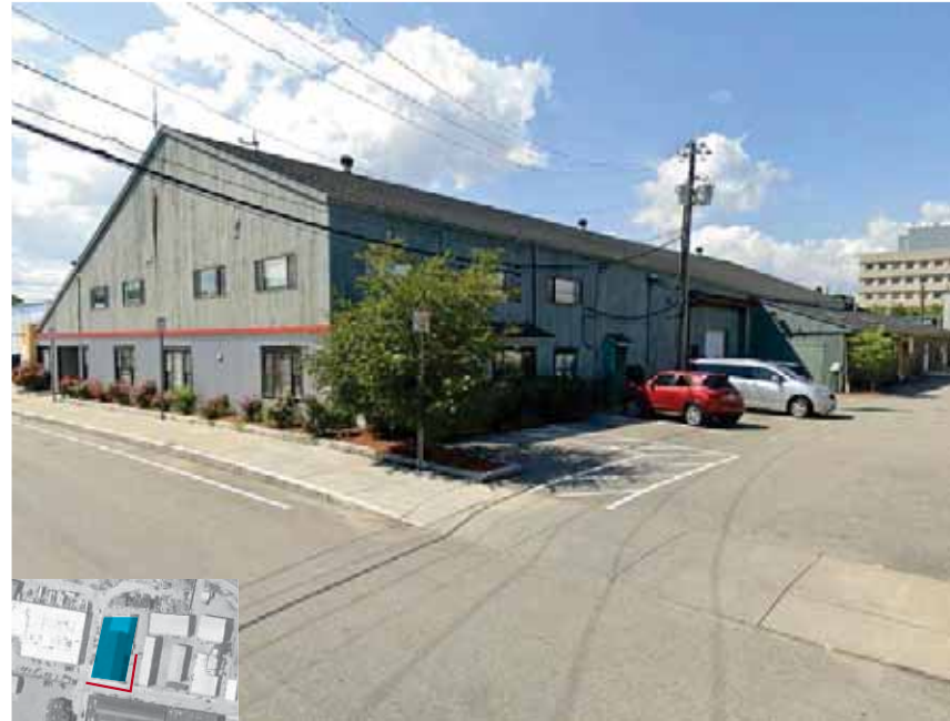
Southeast Corner of Site
