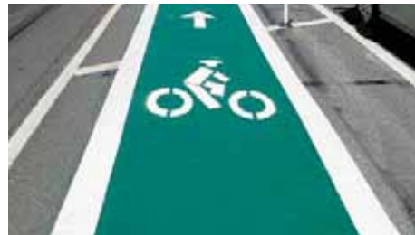
PERMEABLE ASPHALT BIKE PATH
