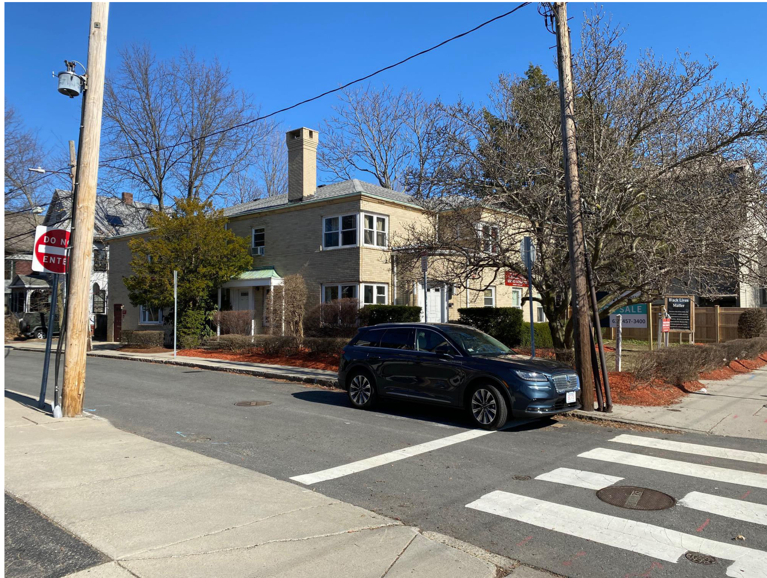
MASS AVE. & MILTON ST. CORNER VIEW
