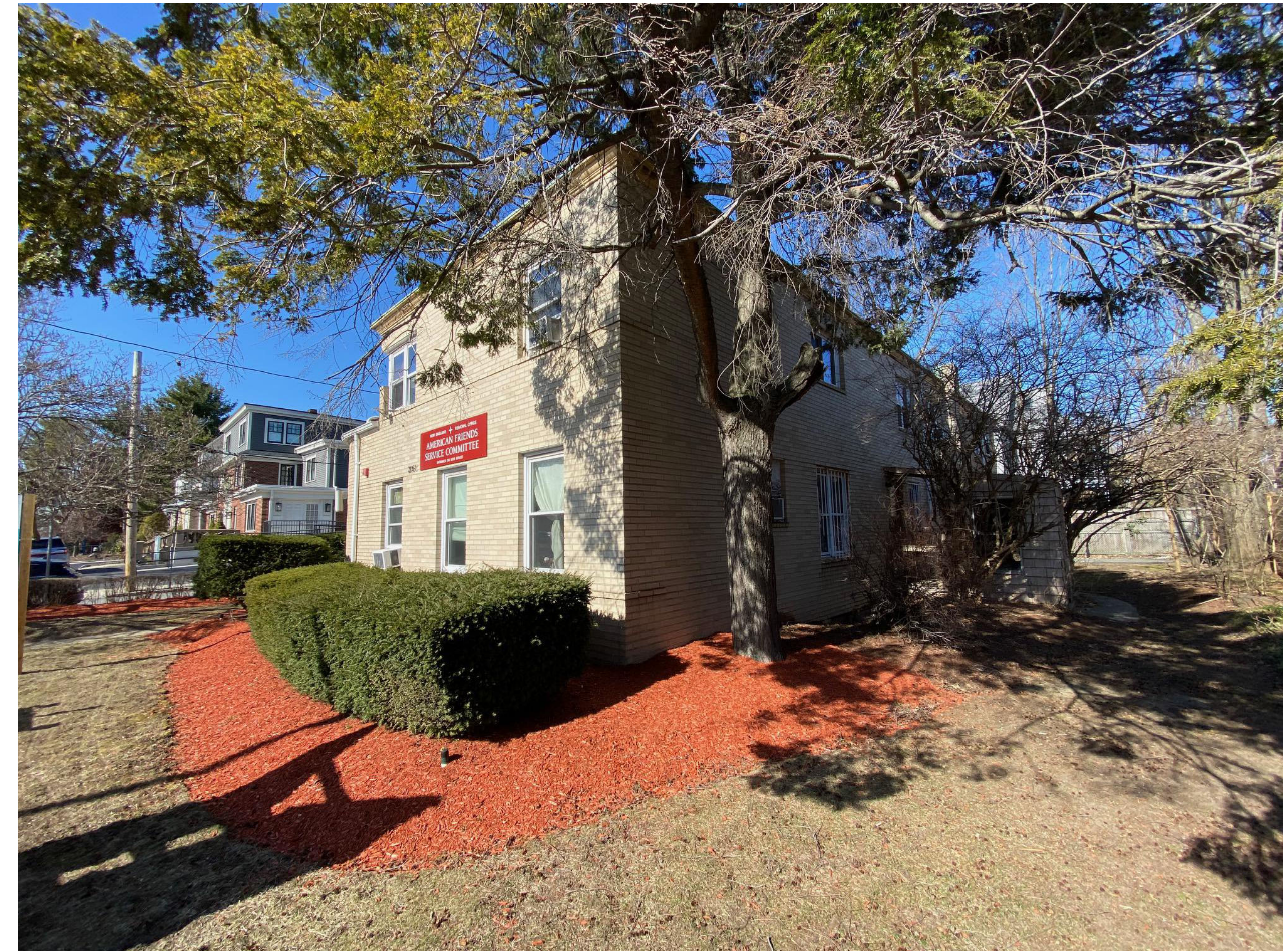
MASS AVE. CORNER VIEW
