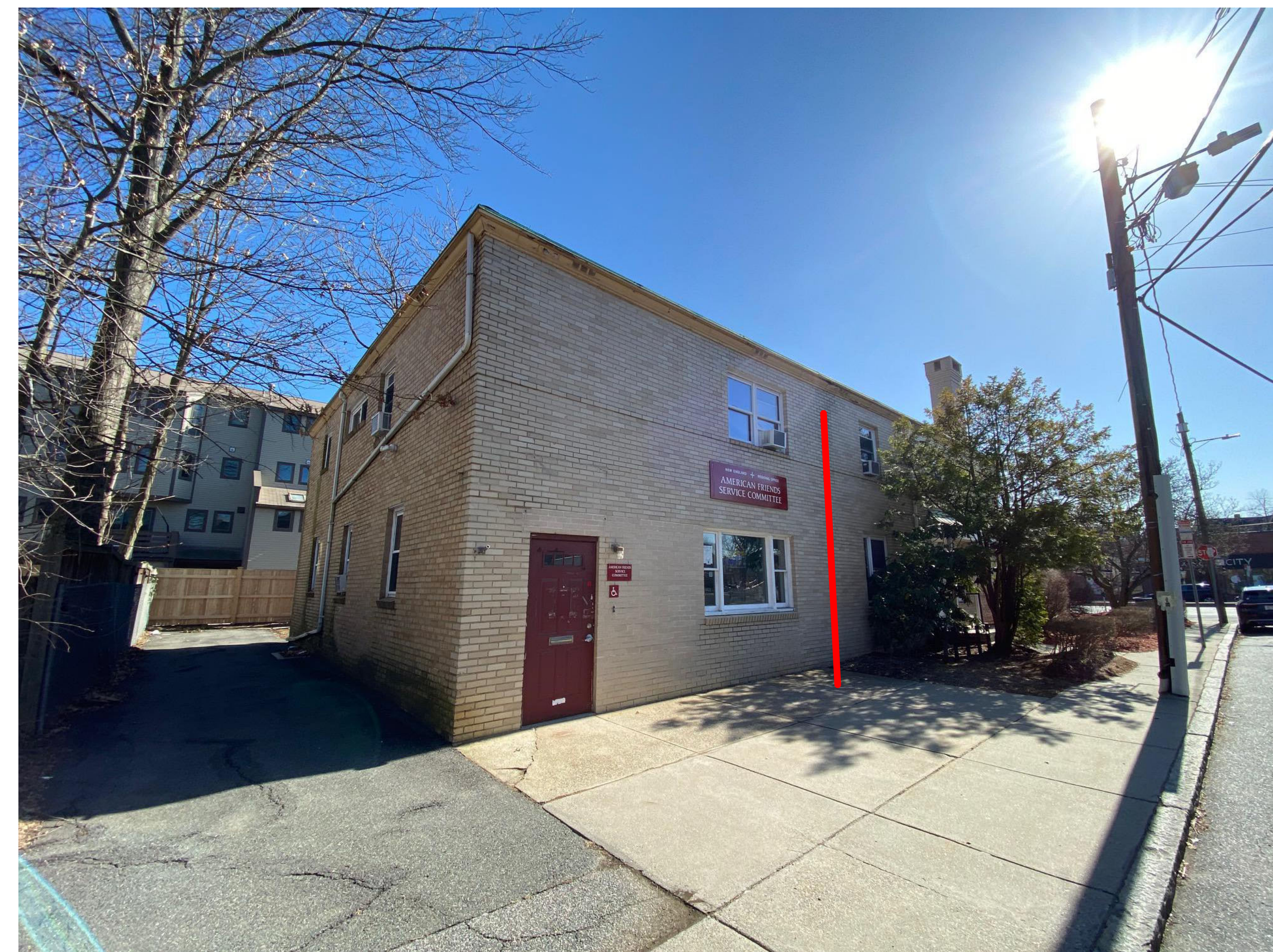
CURRENT, MILTON STREET VIEW
