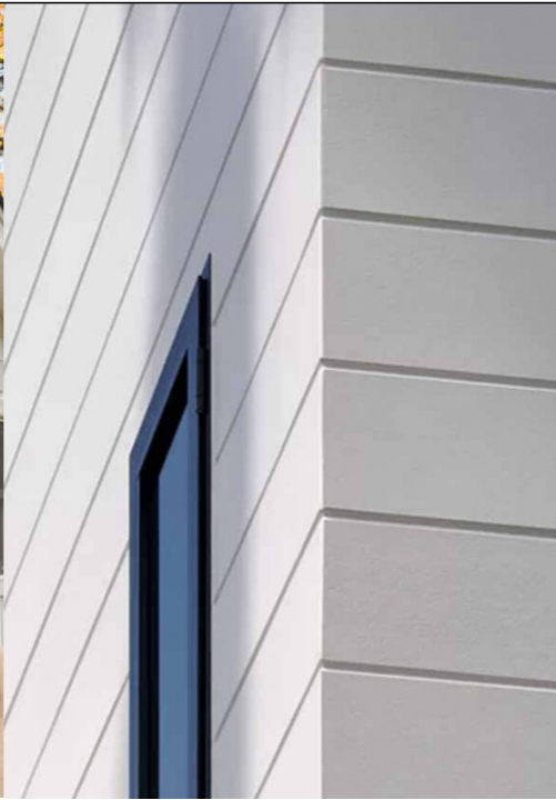
HARDIE PLANK SHIPLAP SIDING ACCENT SIDING (#8 & 10)
