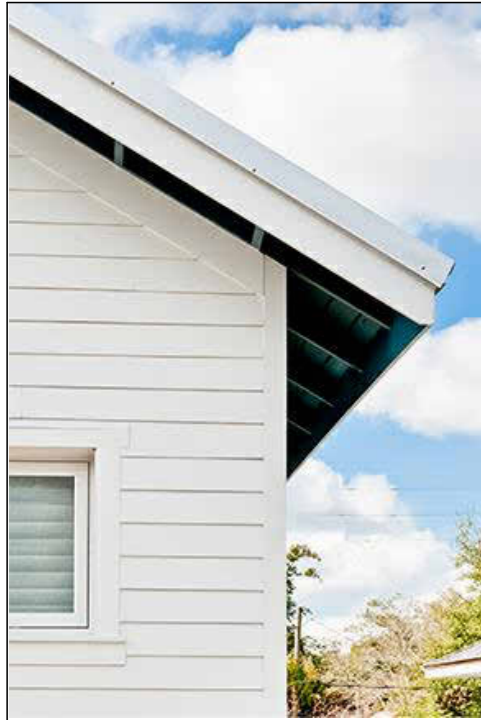
HARDIE PLANK CLAPBOARD SIDING PRIMARY SIDING MATERIAL (#8 & #10)
