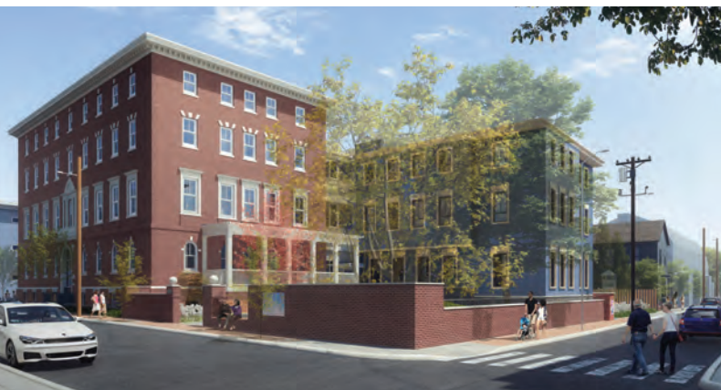
116 Norfolk Street. Construction is underway on 62 affordable rental units with on-site support services for low-income residents.
