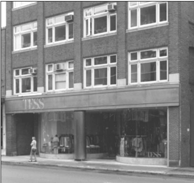
Figure 3. Tess storefront, 20 Brattle Street, 1999.
