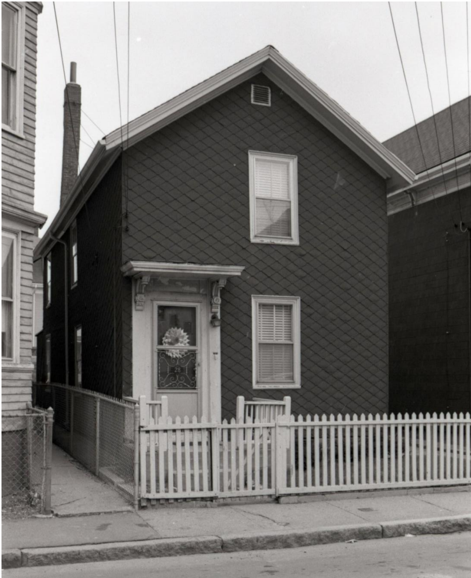
CHC survey photo of 28 Union St. Bonnie Orr, photographer. Winter 1966-67.
