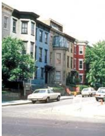
Changing the historic character of the streetscape with additions to rooftop and bay.
