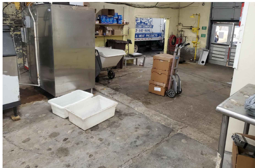
MIDDLE BUILDING EXISTING FLOOR SLABS
