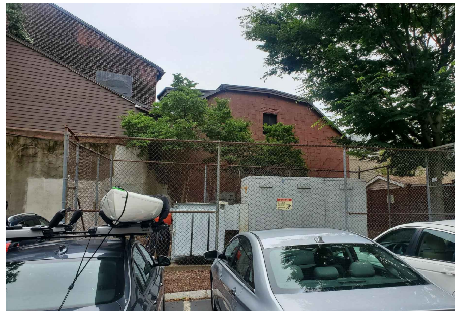
REAR ELEVATION EXISTING CONDITIONS- BARN AND MIDDLE BUILDING
