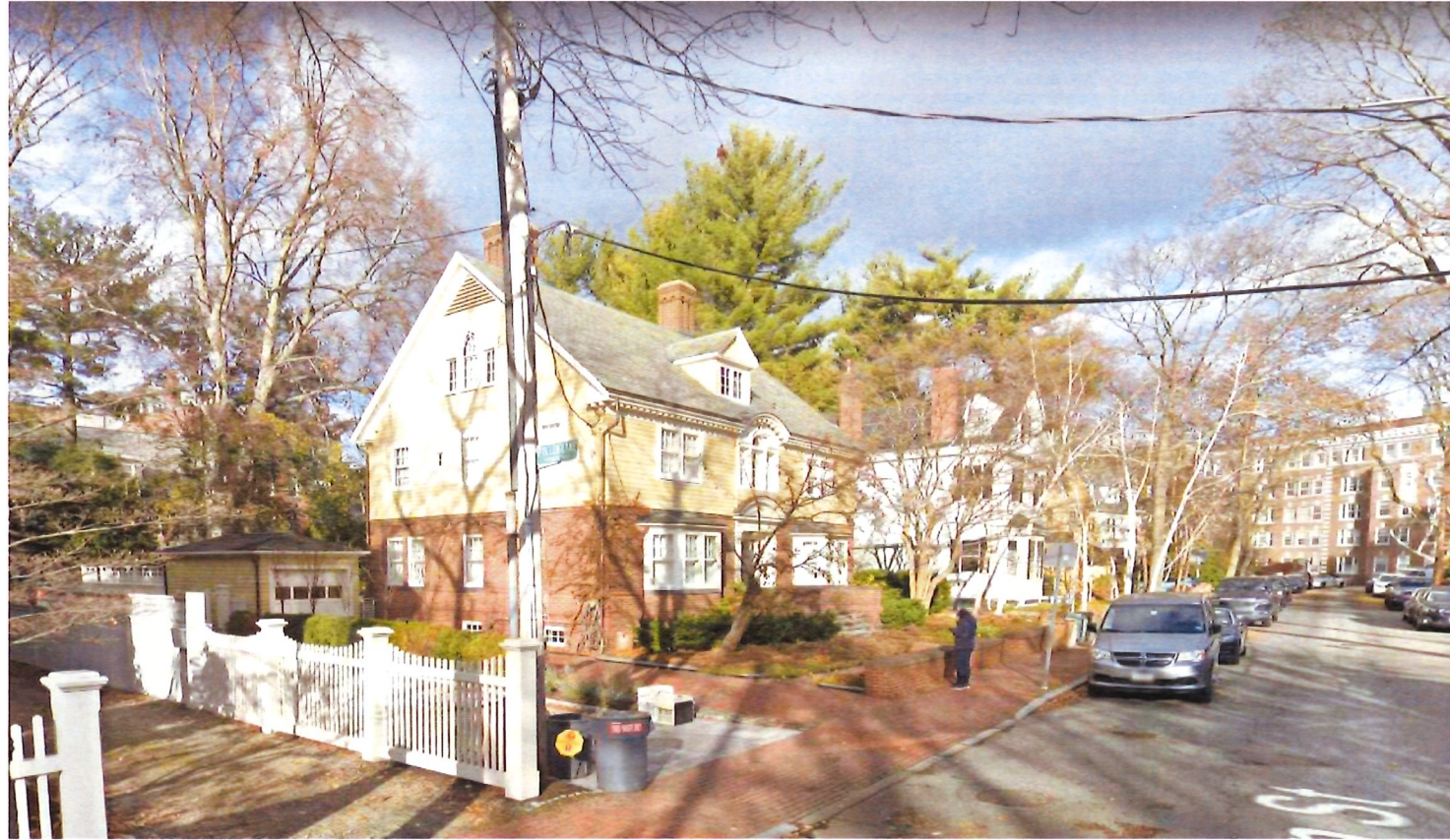
15 FOLLEN - VIEW FROM STREET LOOKING RIGHT
