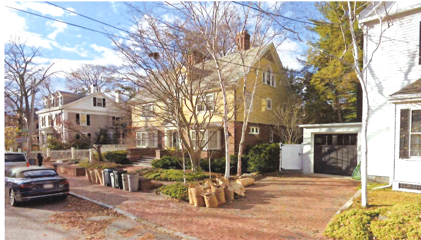
15 FOLLEN - VIEW FROM STREET LOOKING LEFT
