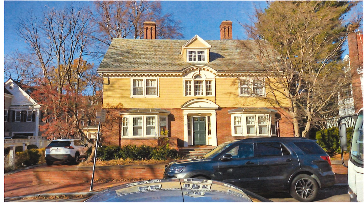
15 FOLLEN- STREET FACADE (FRONT)
