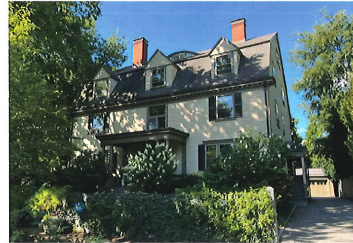
VIEW FROM SIDEWALK LOOKING WEST
