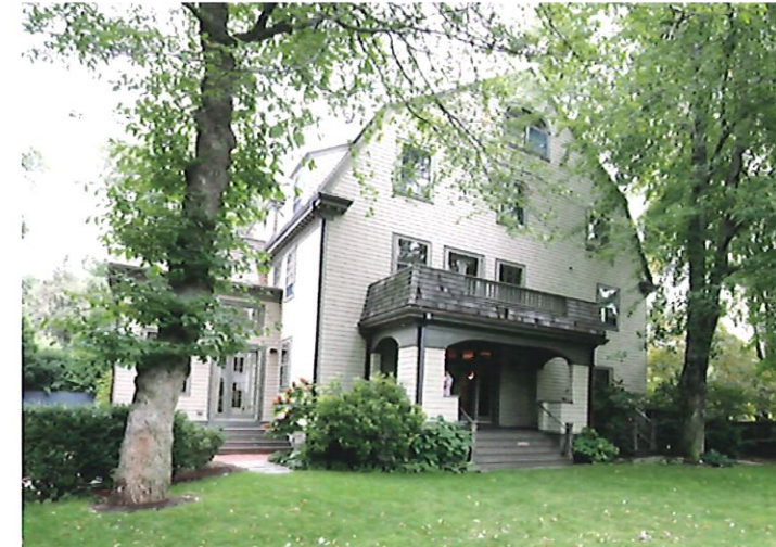
VIEW FROM SIDE YARD LOOKING NORTHEAST
