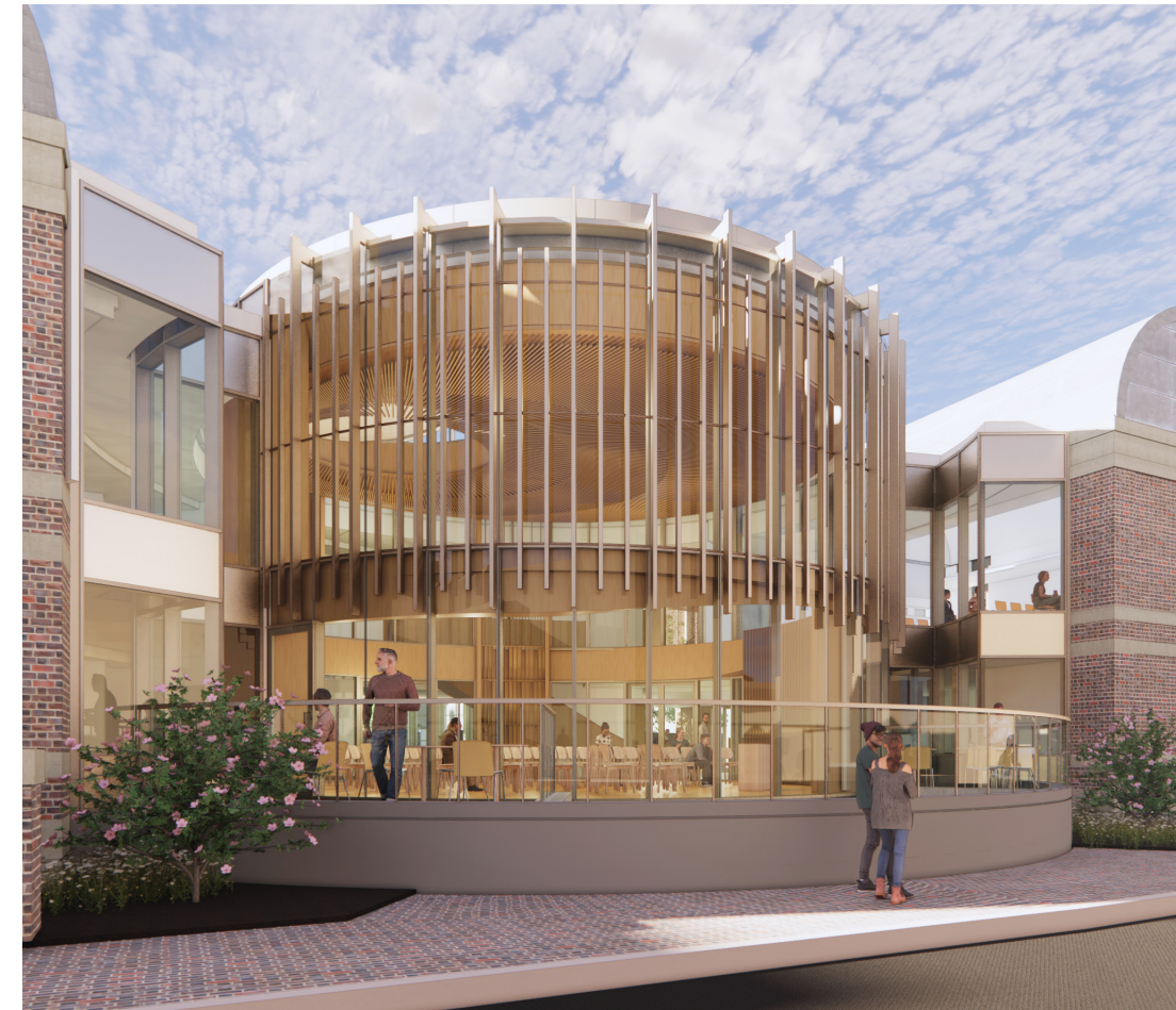
COURTYARD ENCLOSURE (CAST STONE SITE WALL, METAL AND GLASS CURTAINWALL, PAINTED METAL VERTICAL SUN SHADES)
