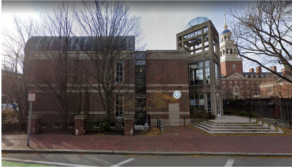
NORTH FACADE FROM MOUNT AUBURN STREET - EXISTING
