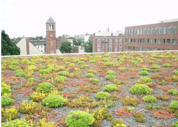
Green Roof at 23 Sidney Street University Park - Credit: Cambridge Community Development
