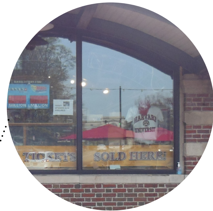
restore glass and frames
