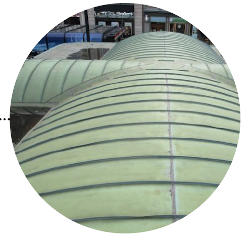
standing seam copper roof
