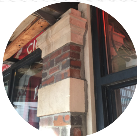
masonry and limestone piers
