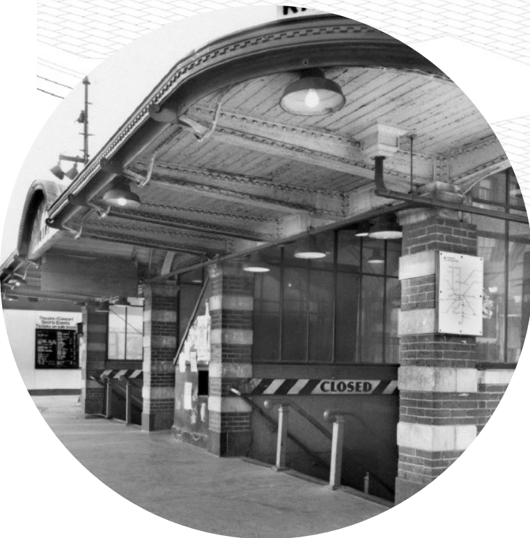
original entrance into train
