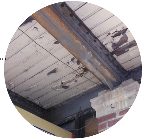
riveted iron structure & exposed wood beadboard
