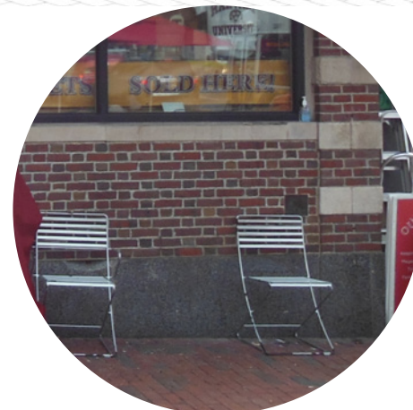
perimeter brick wall with granite base
