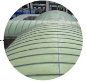
standing seam copper roof
