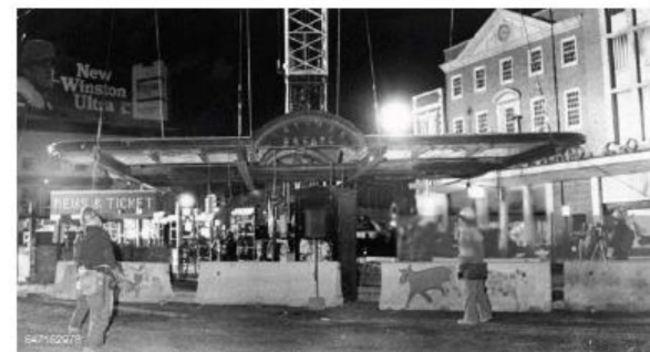
moving of kiosk roof & structure (photo credit: Boston Globe)
