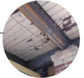
riveted iron structure & exposed wood beadboard
