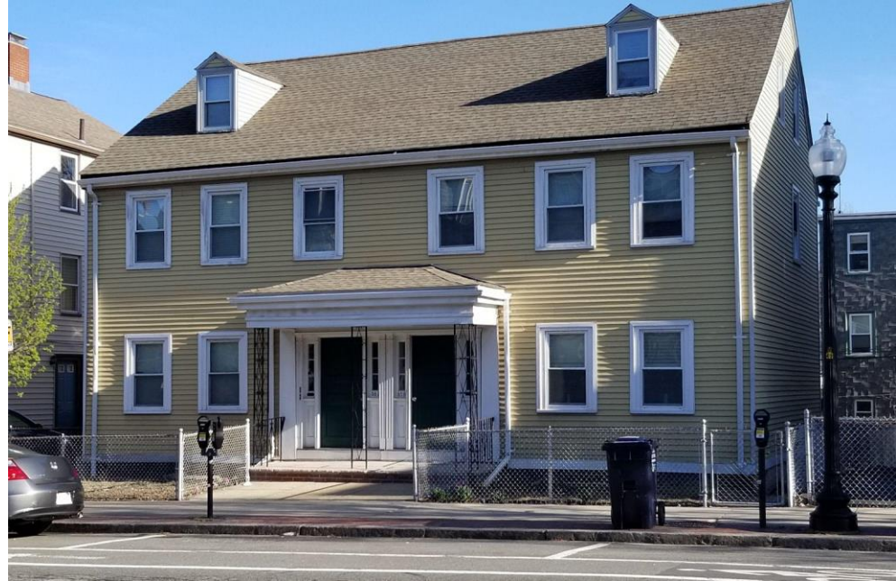
Existing housing structures on Cambridge Street.
