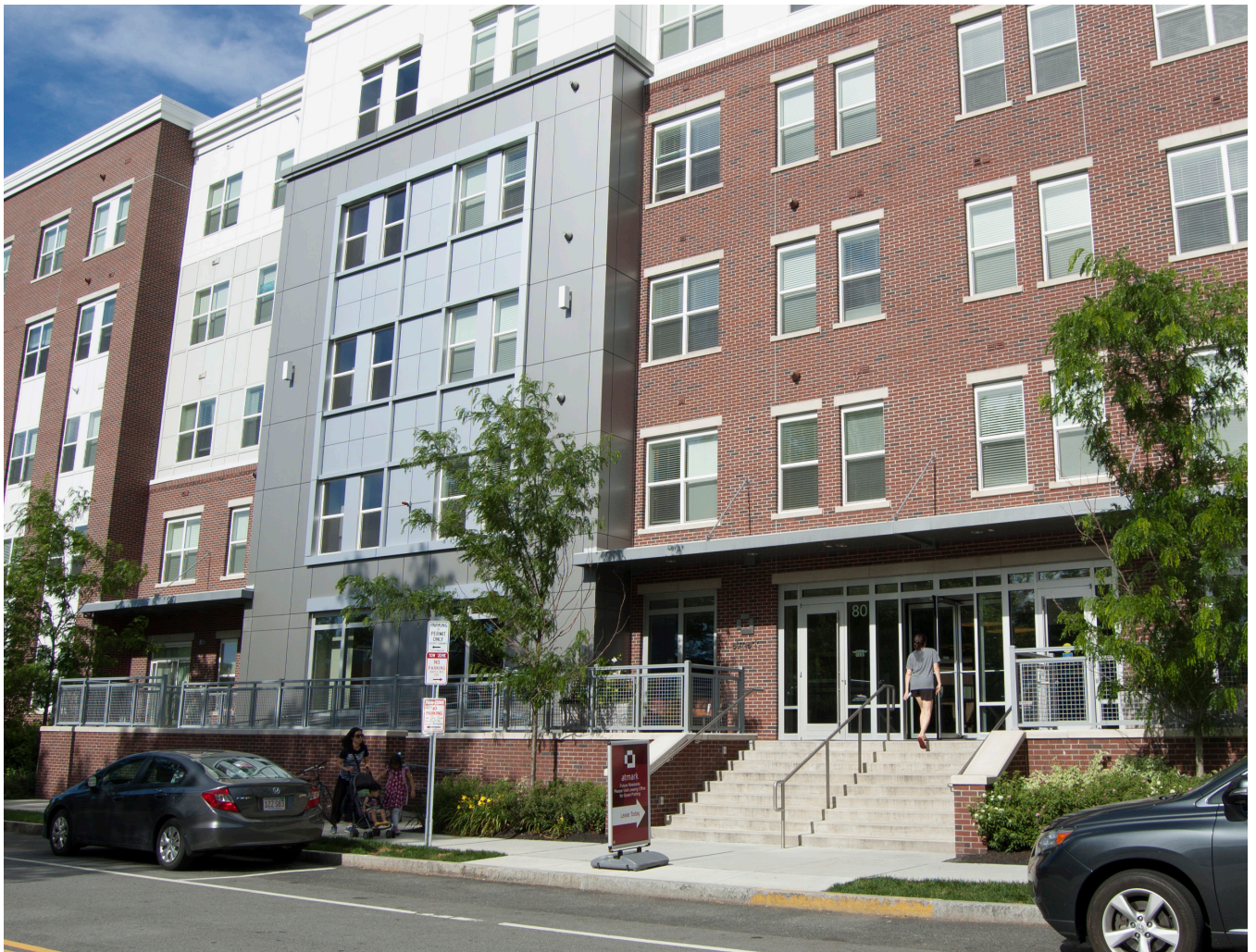
An elevated first floor is one design feature meant to protect occupants from flooding.
