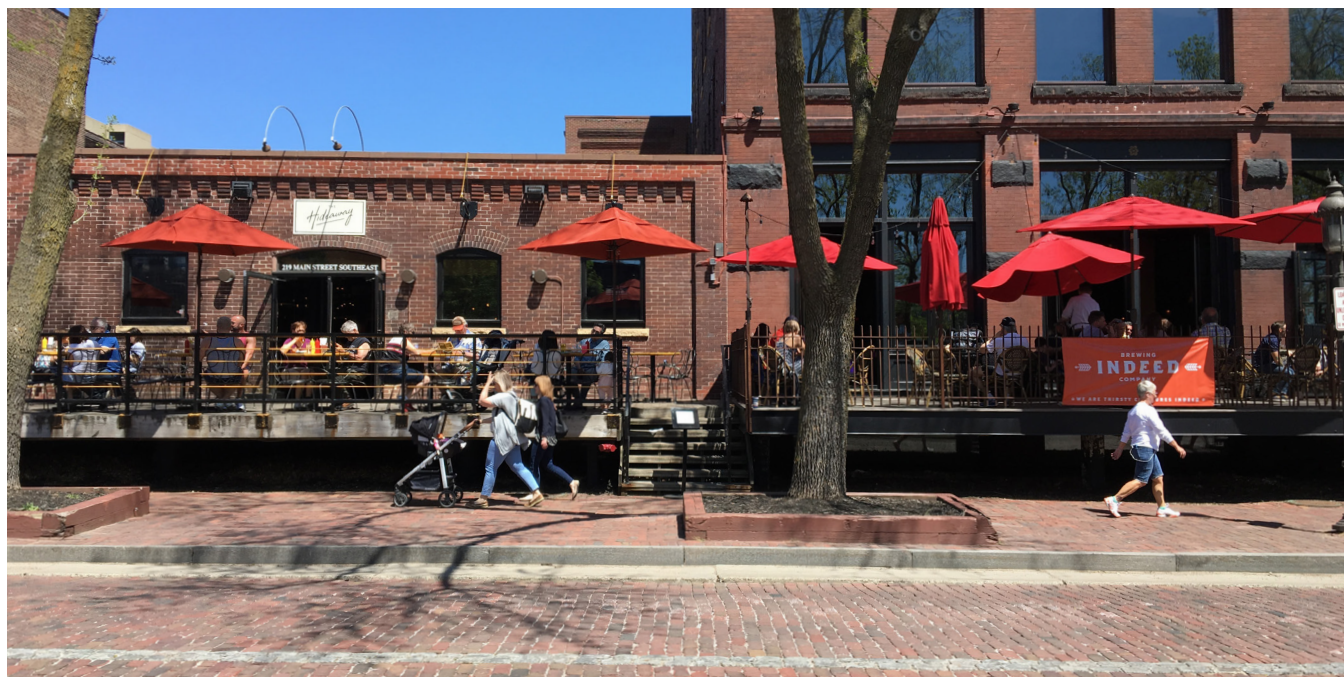
An elevated walkway will provide a secondary public realm as a result of raising the first floors of buildings to protect from future flooding.
