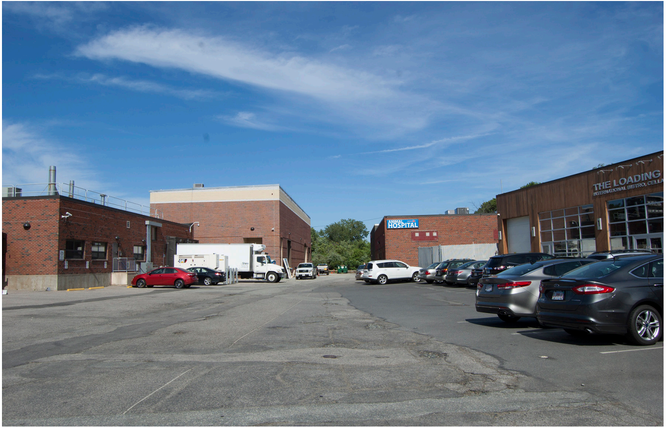
Single-story office and industrial buildings surrounded by parking exemplify the overall low building densities found in Alewife.
