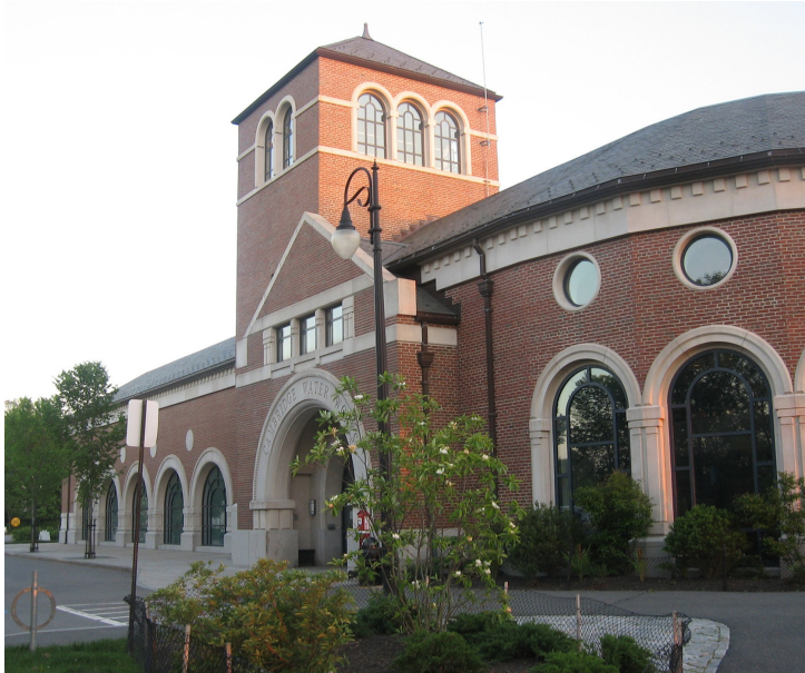
The Walter J. Sullivan Water Purification Facility sits on Fresh Pond and services all of Cambridge.
