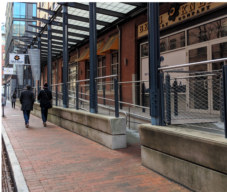
Elevated walkways are increasingly common today in potential flood zones, like Boston's Fort Point Neighborhood above.
