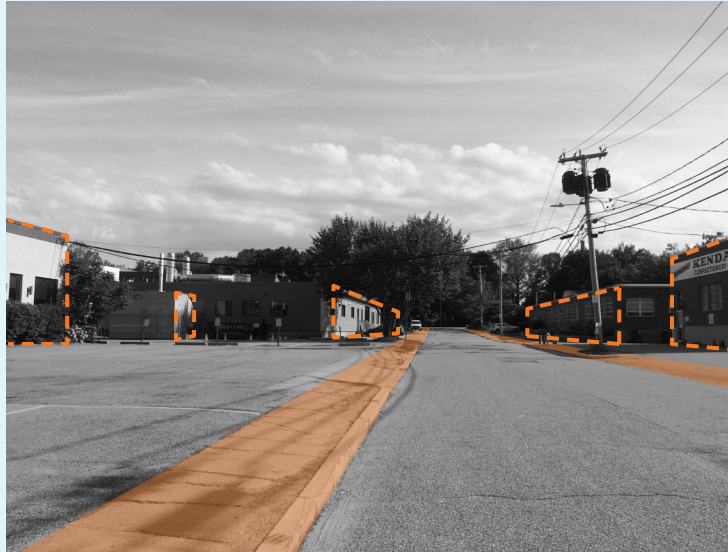
Buildings in Alewife are often disconnected and set back from the street. Streets without a well-defined street wall can be less enjoyable to walk on.
