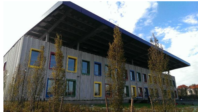
Contiguous Panels Mounted on Structure above Roof
