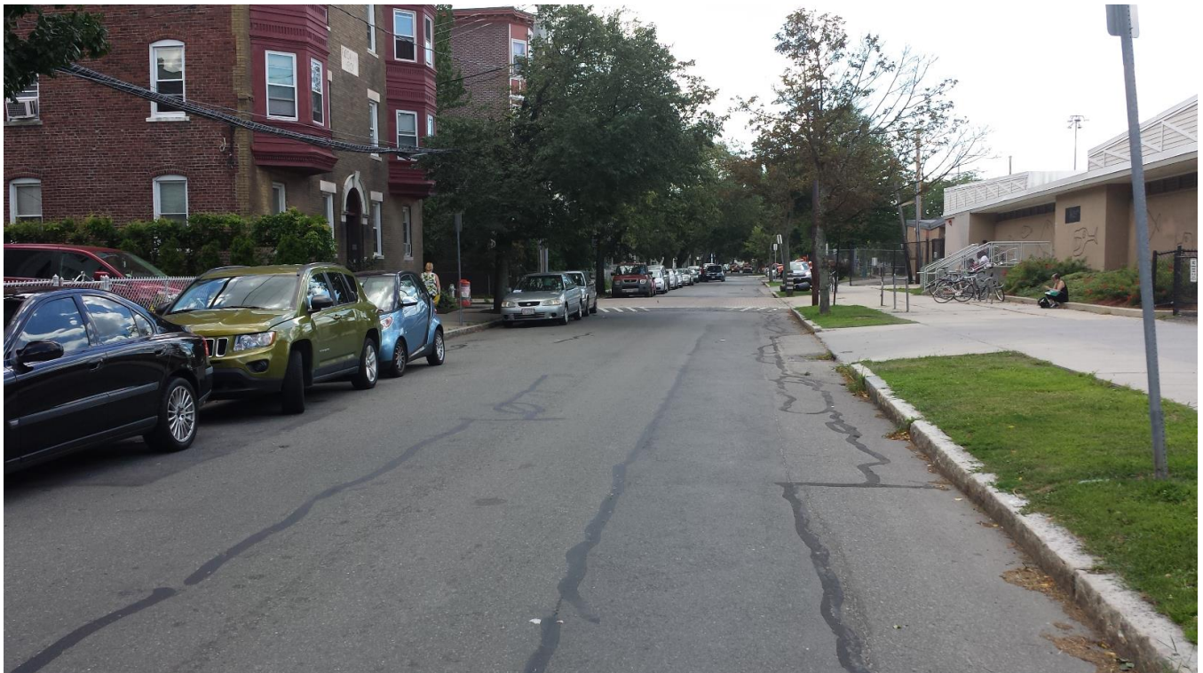
PHOTO 4: VIEW SOUTHBOUND FROM CAMBRIDGE STREET
