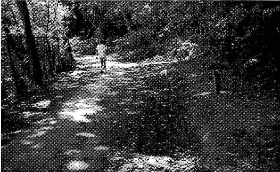
Figure 16: Soil Erosion and Compaction, Perimeter Road, 1998 Source: Rizzo Associates, Inc., Summer 1998
