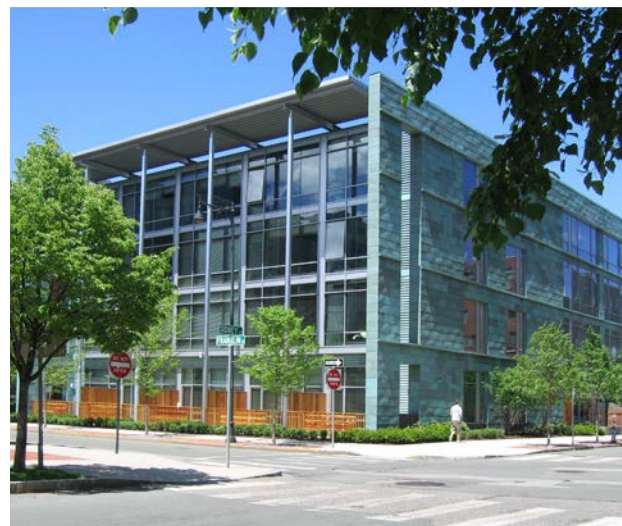
Emphasize the civic importance of primary public spaces by differentiating between principal front facade and side facades by means such as contrasting materials, colors, scales, the amount and type of detail and articulation, and compositional formality vs. informality.
