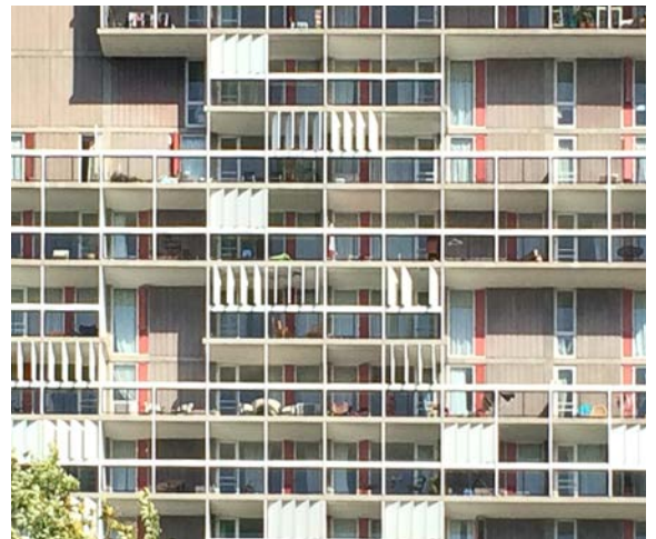
Balconies and sun shading devices can add visual interest.
