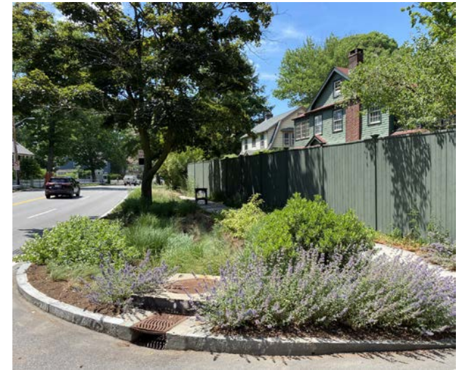
Rain garden / bioswale on Fresh Pond Parkway at Larch Rd.
