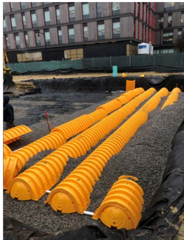
Stormwater infiltration system installed under new Toomey Park in East Cambridge.
