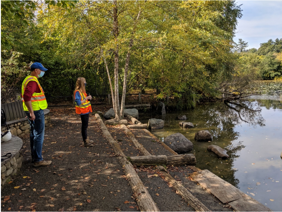
SHORELINE CONDITIONS WITH DESTABILIZED LOG AND GRANITE CURB EDGING (2020)
