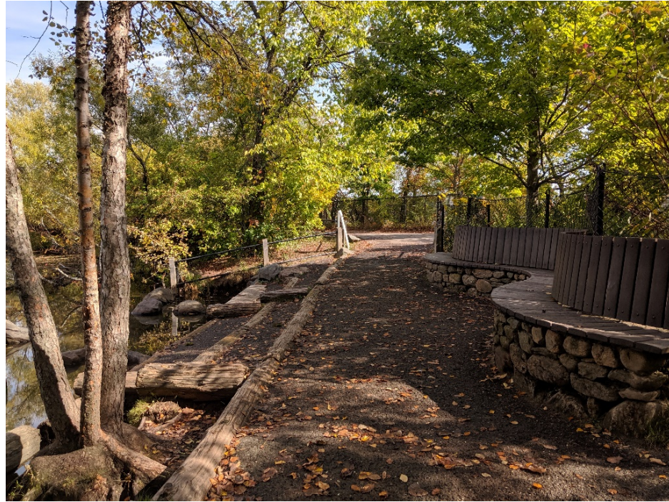
SHORELINE CONDITIONS WITH DESTABILIZED LOG AND GRANITE CURB EDGING (2020)
