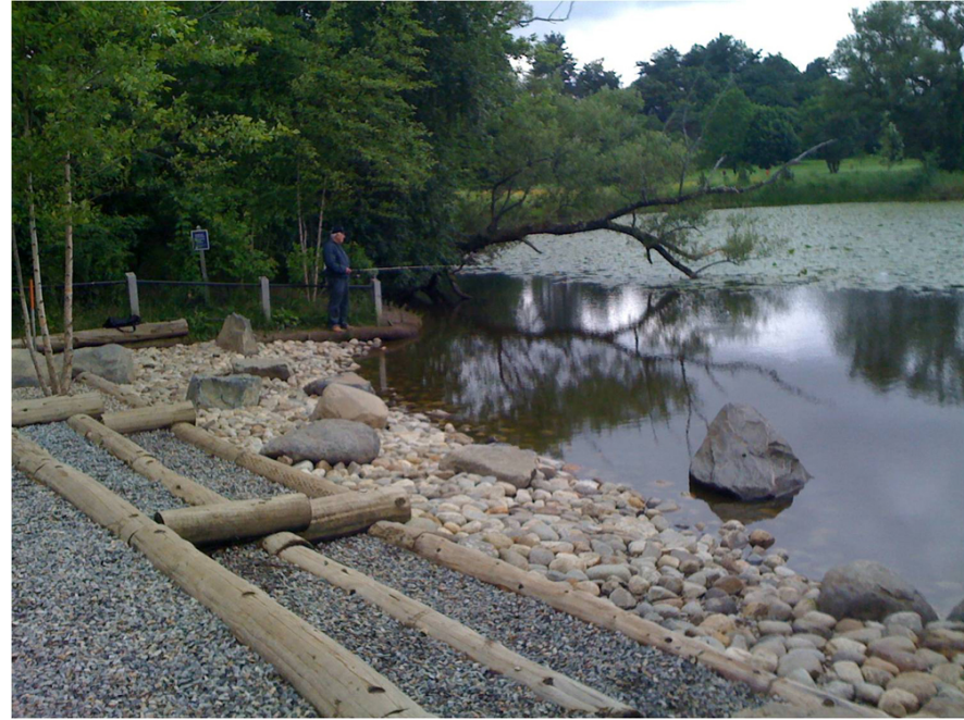
PHOTO OF NEWLY CONSTRUCTED SHORELINE (2007)
