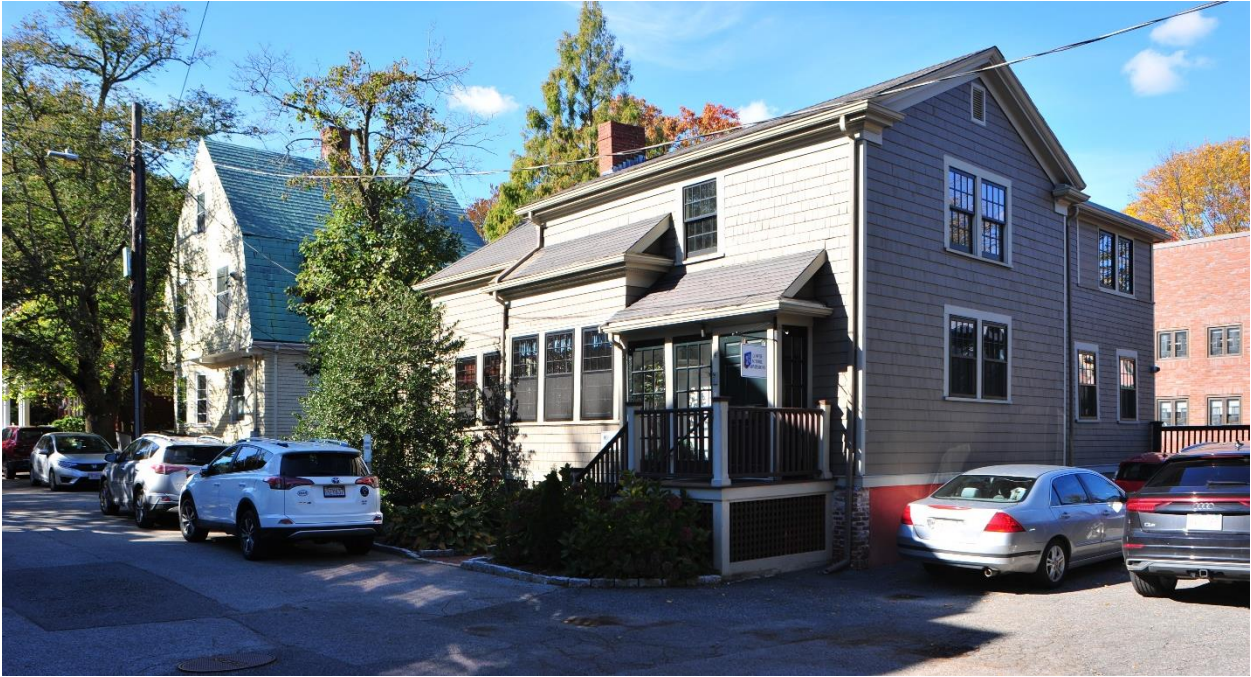
South and east elevations of 6 Buckingham Place. Two-story addition at right. CHC staff photo, Nov. 2021.
