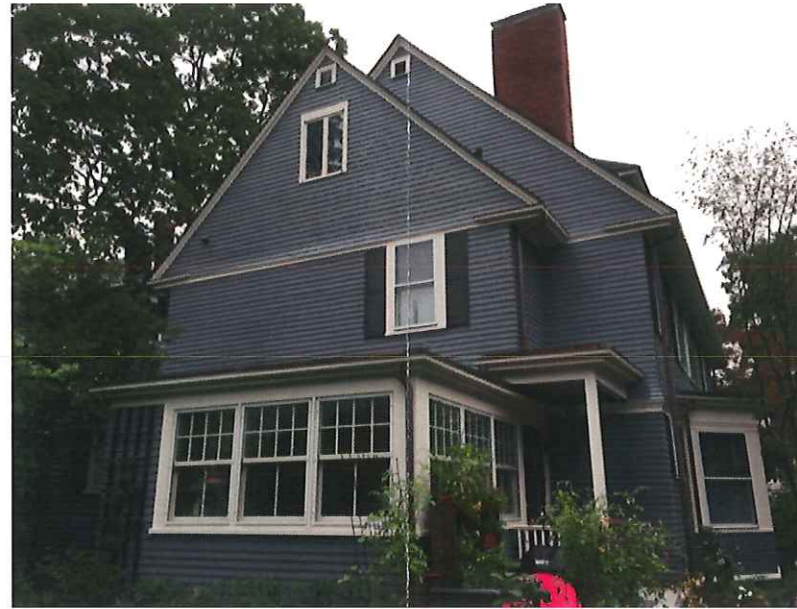
② VIEW OF EXISTING REAR AND LEFT SIDE ELEVATIONS
