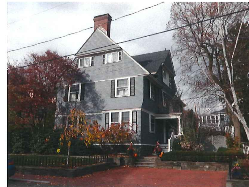
⑥ VIEW OF EXISTING FRONT ELEVATION
