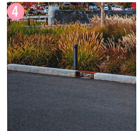
BITUMINOUS CONCRETE PAVING
