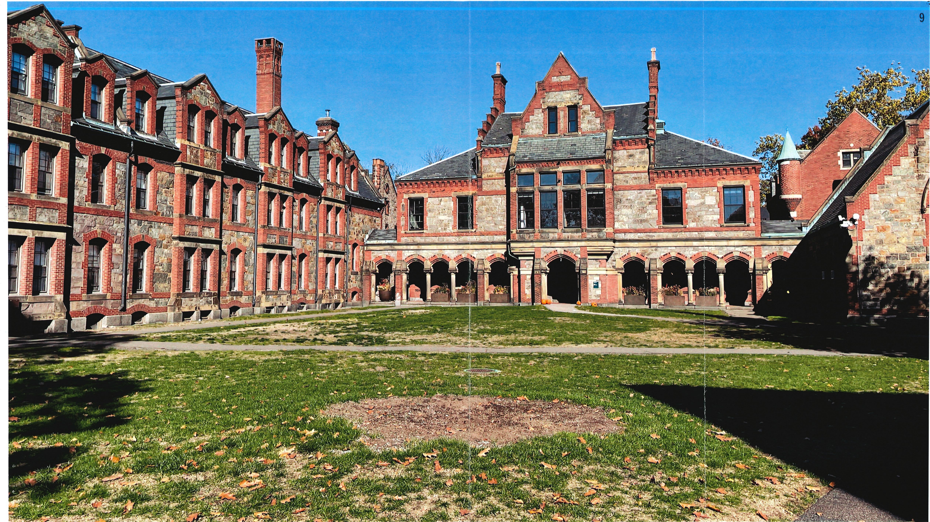
SOUTH CAMPUS | EXISTING VIEW OF REED HALL AND QUAD
