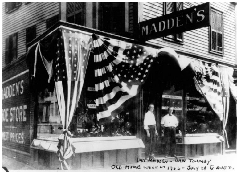
635 Cambridge Street (1867) with new storefront, 1906 CHC
