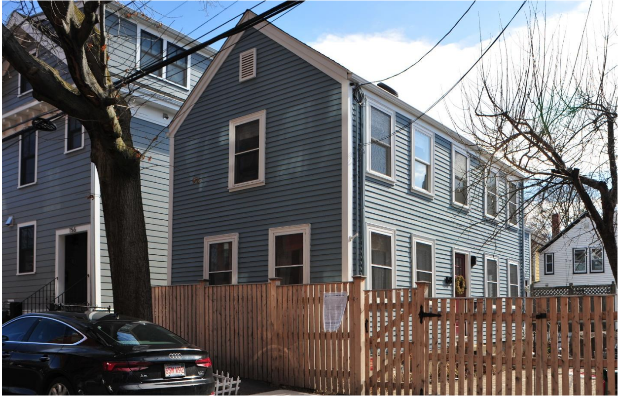
158 Thorndike Street before renovation.
