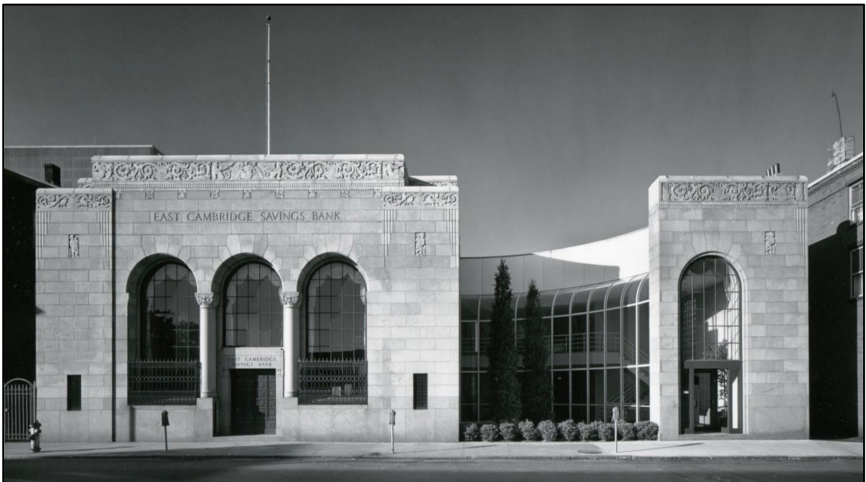
East Cambridge Savings Bank, constructed in 1931 (left), with 1977 addition (right) Steve Rosenthal photo, CHC
