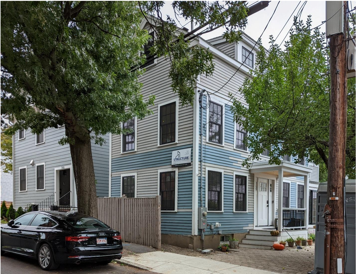
158 Thorndike Street, with renovation in process.
