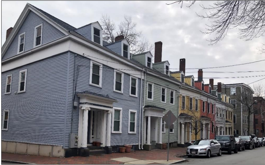
Greek Revival rowhouses (1842) at 36-46 Second Street
