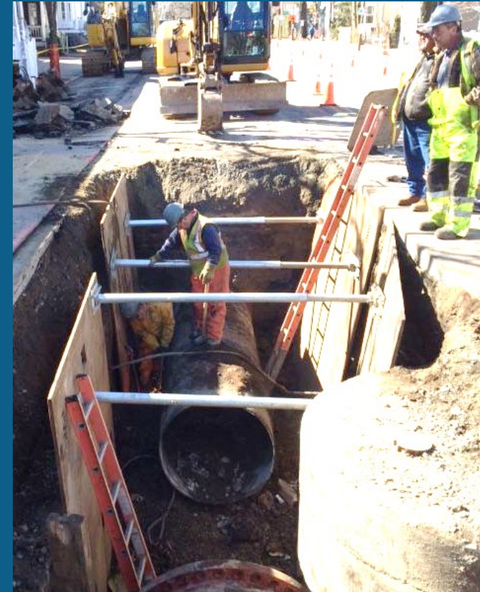
Upgrades to affected utilities
