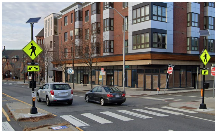
Rectangular Rapid Flashing Beacon (RRFB)
