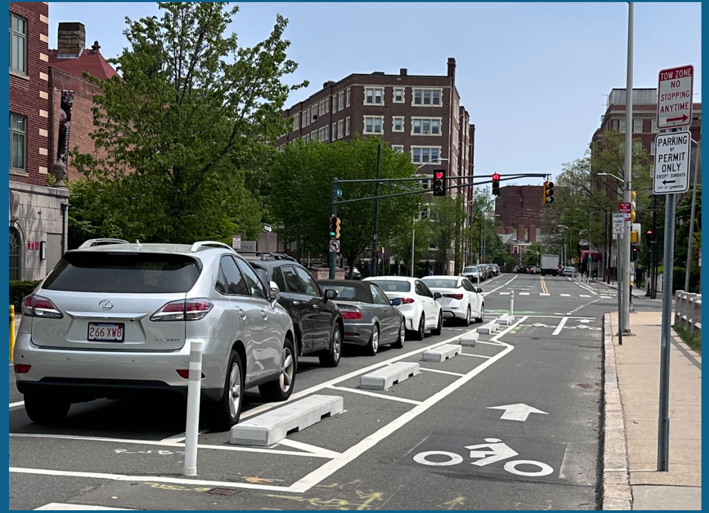
Curbed bike lane separation
