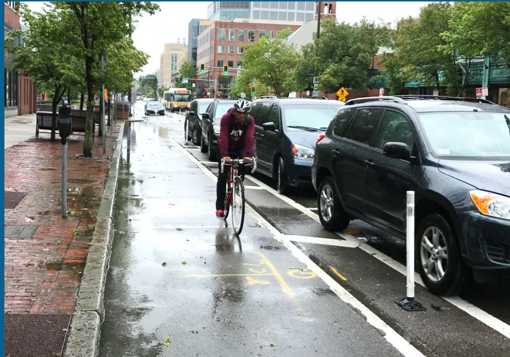
Flex post bike lane separation
