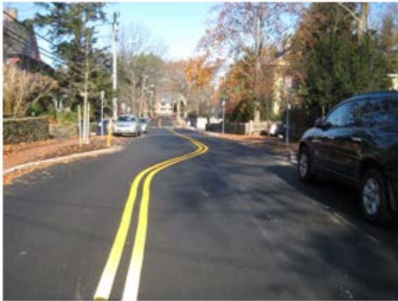
Street with Traffic Calming
