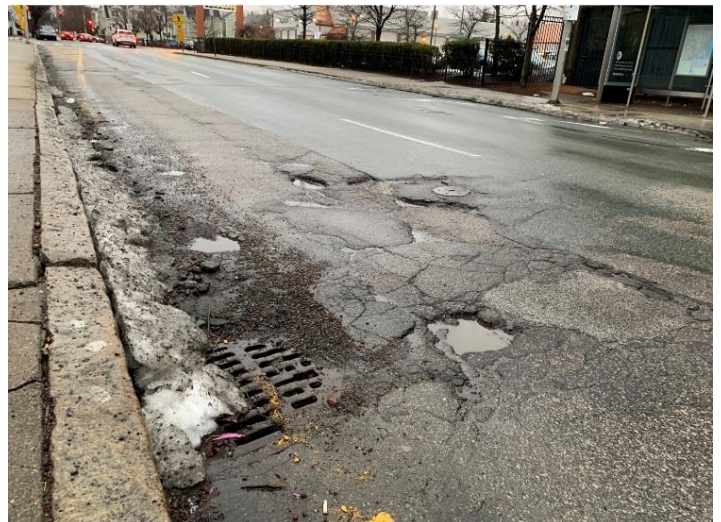
Figure 4: Existing Vehicular Infrastructure
