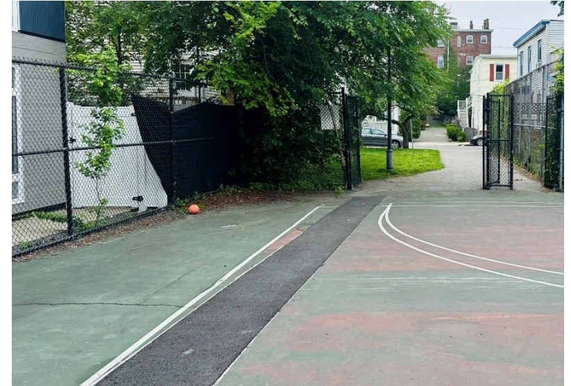
Runoff Pavement at Fencing
