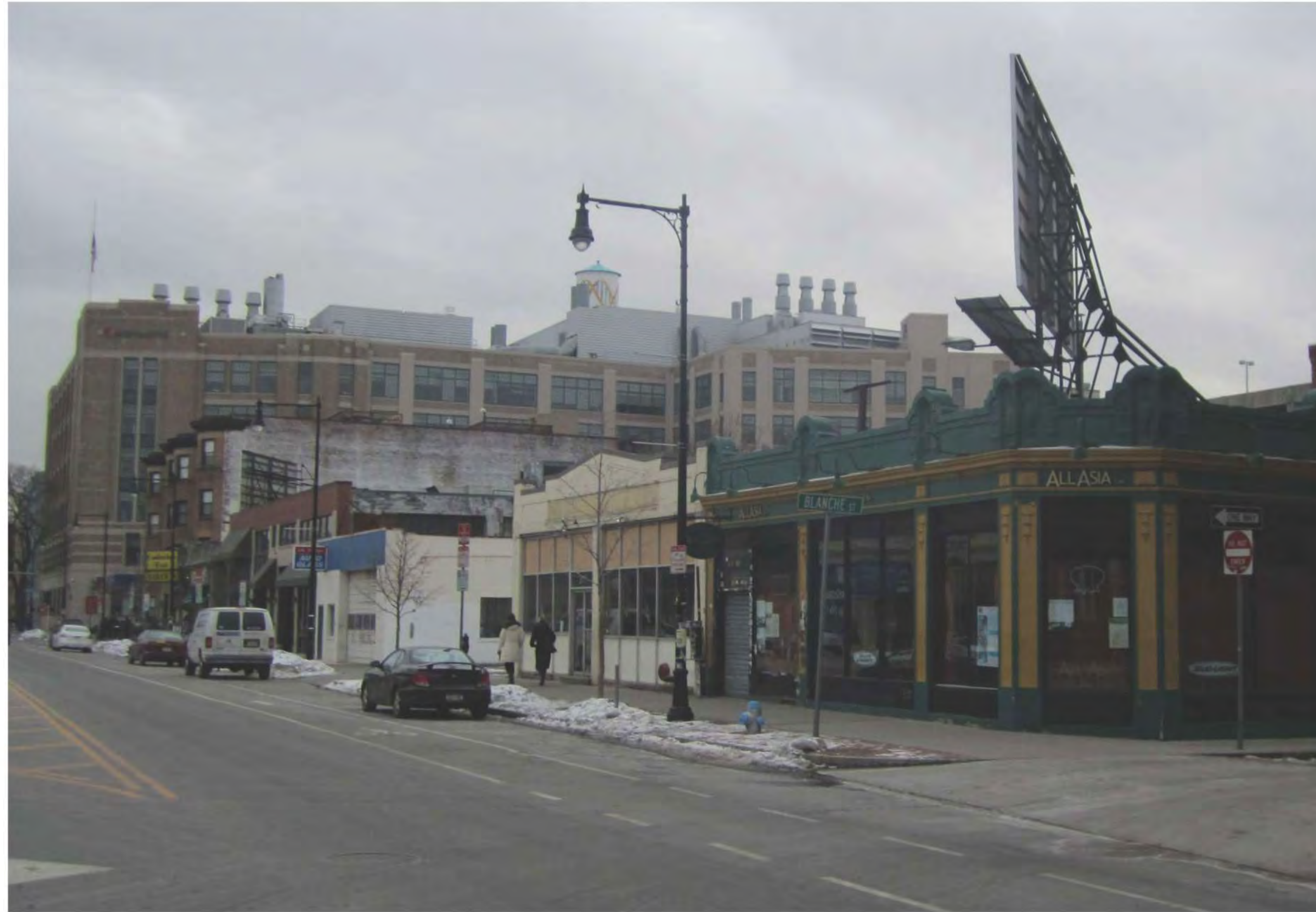
Existing Conditions CORNER OF MASS AVE AND BLANCHE STREET
