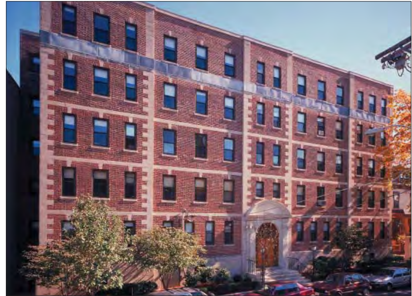
Existing Conditions - 20-20A Prescott Street
