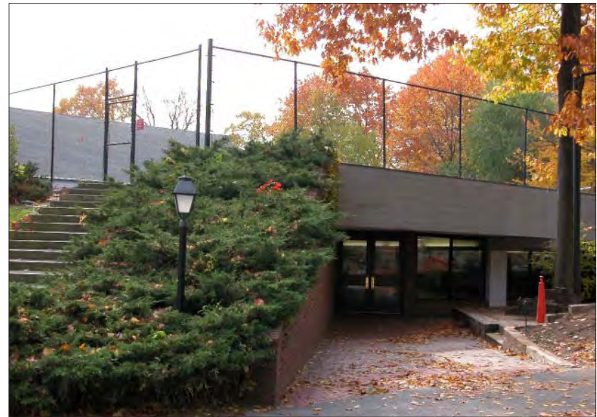
Quadrangle Athletic Facility
