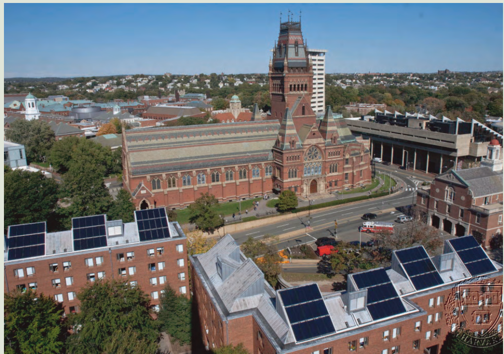
The new solar thermal installation on the roof of Canaday Hall is one of many alternative energy projects at Harvard.
