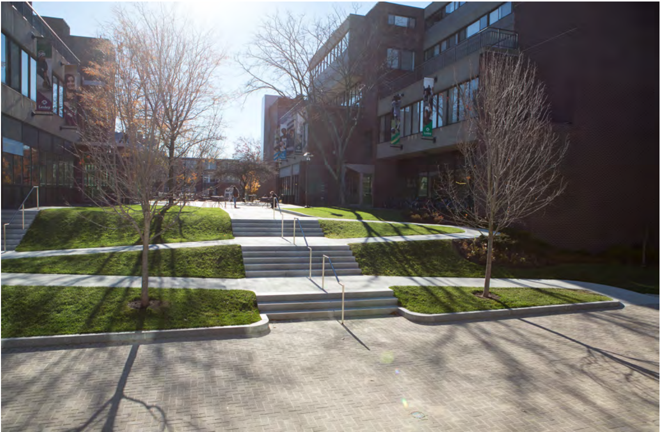
THE NEW PEDESTRIAN WAY IMPROVES STORMWATER MANAGEMENT AND ACCESSIBILITY.
