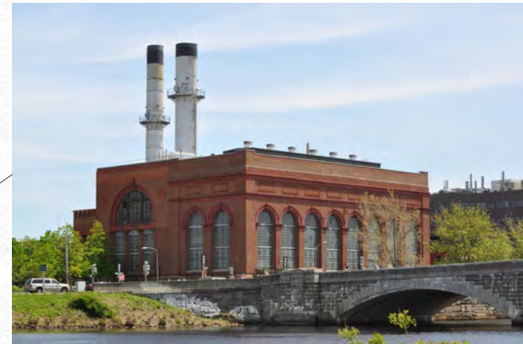
Blackstone Steam Plant
