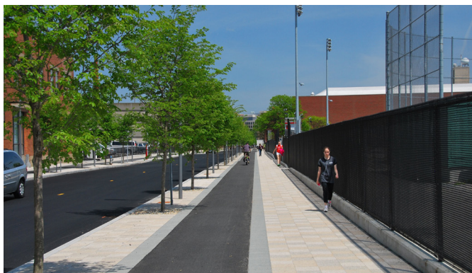
Vassar Street with a fully grade-separated bicycle facility.
