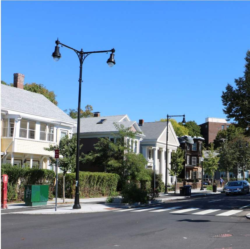
Roadway Lighting ( Western Ave )
