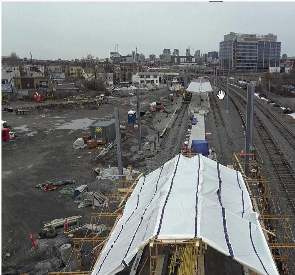
Station under construction at Union Square
