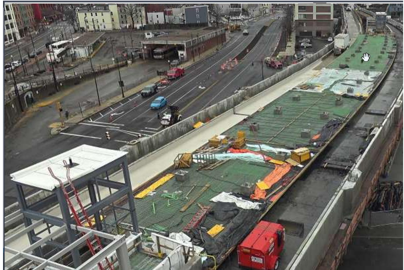
(New) Lechmere Station under construction
