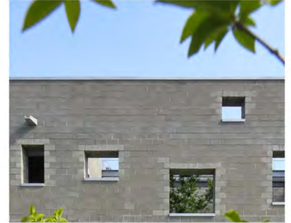
Perforated Masonry Wall
