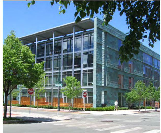
Emphasize the civic importance of primary public spaces by differentiating between principal front facade and side facades by means such as contrasting materials, colors, scales, the amount and type of detail and articulation, and compositional formality vs. informality.
