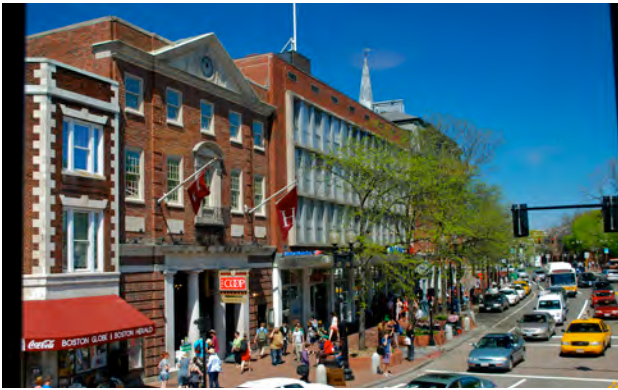
The framing of public space by streetwall facades provides a sense of spatial enclosure.
