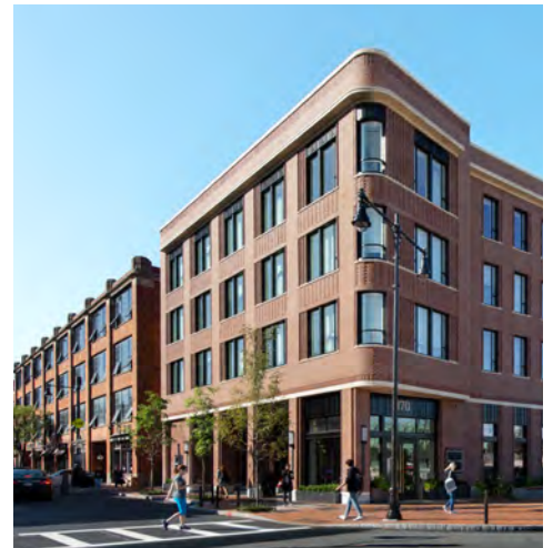
Emphasized corner helps frame the primary street by reinforcing the importance of the facade that addresses it.
