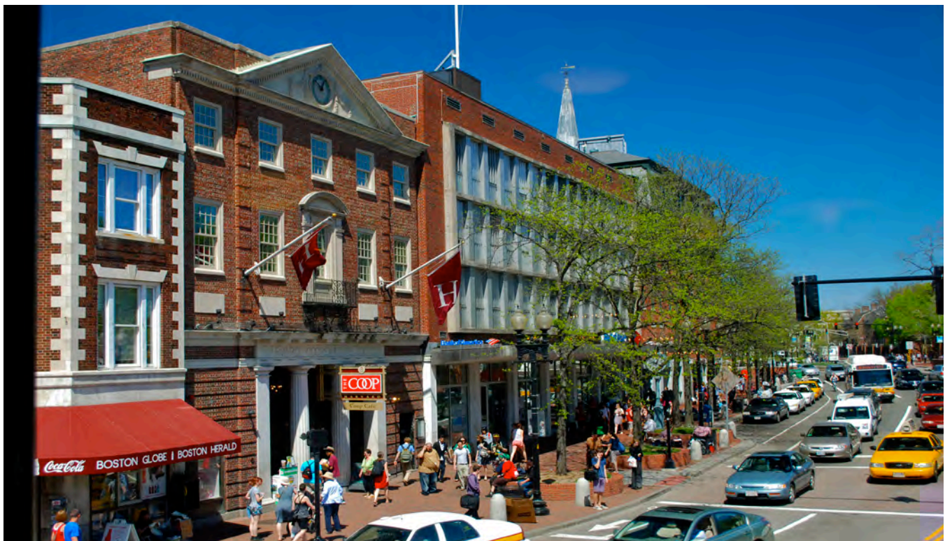
Continuous streetwalls define streets and public spaces. Varied facades visually enrich the streetwall.
