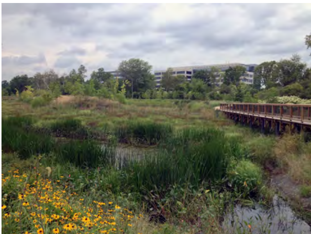
Stormwater mitigation features should be integral parts of landscape design. The Alewife Constructed Wetland is an example.
