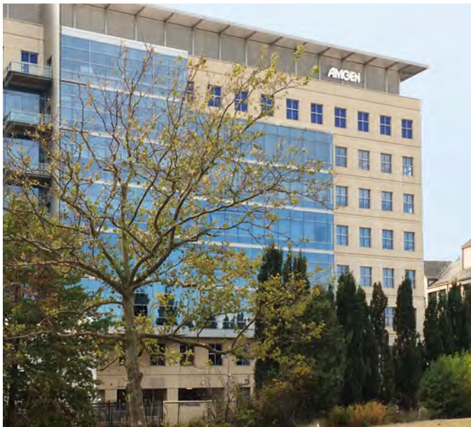
Mechanical equipment and screening should be integral parts of office building design.
