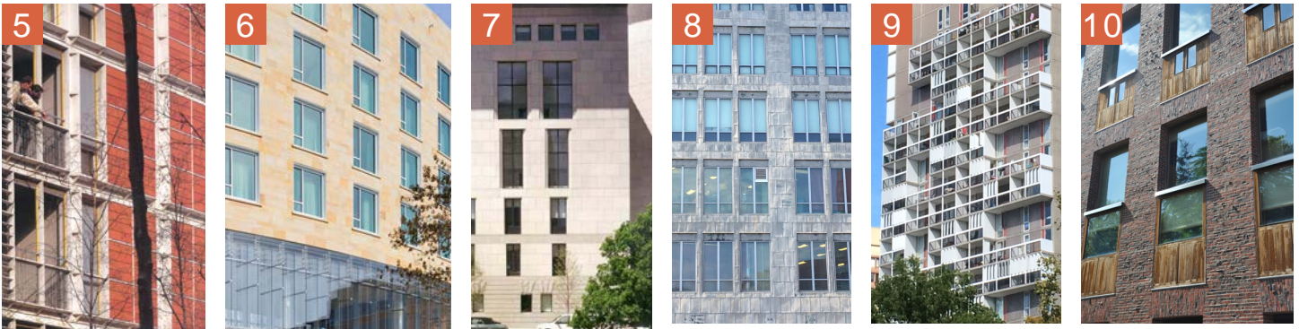
5 - 10. Facade detail, proportion, color, three dimensional relief, and materials should contribute to a rich visual environment.
