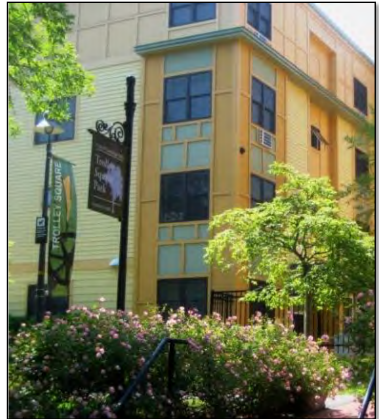
Trolley Square: 40 affordable rental and ownership units
