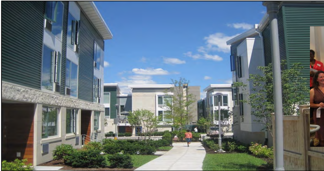
Lincoln Way: 70 reconstructed public housing units
